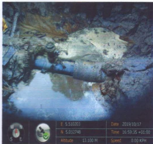
6" valve installed on the line
